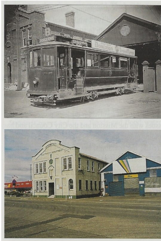
The Invercargill M.E.D. building and tram barn which are to be preserved.
